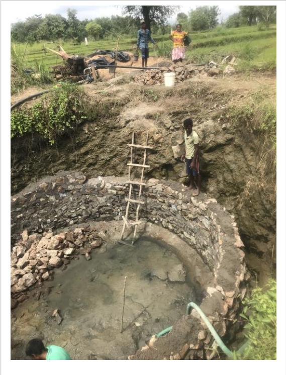
Construction of agro-wells at Veheragala (left) and Sulugune (top and bottom)
